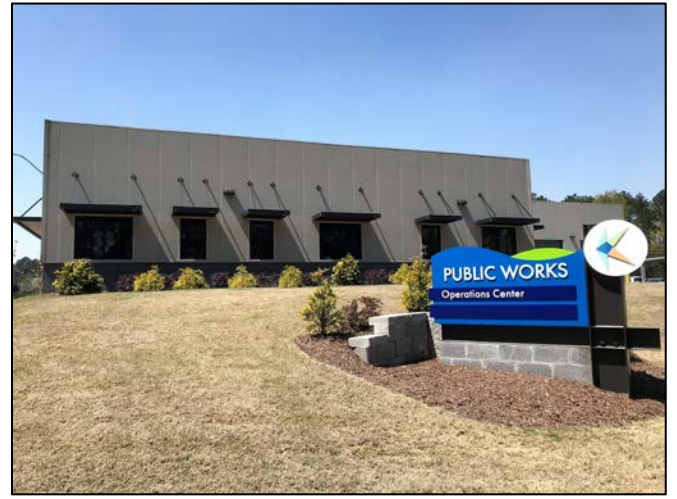
Public Works Facility
