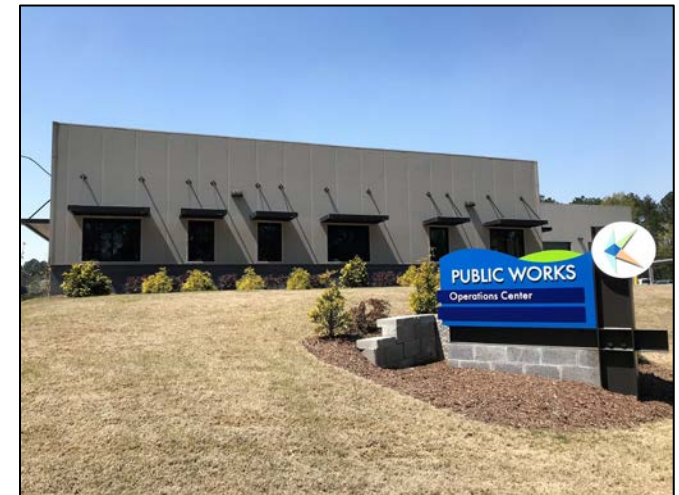
Public Works Facility
