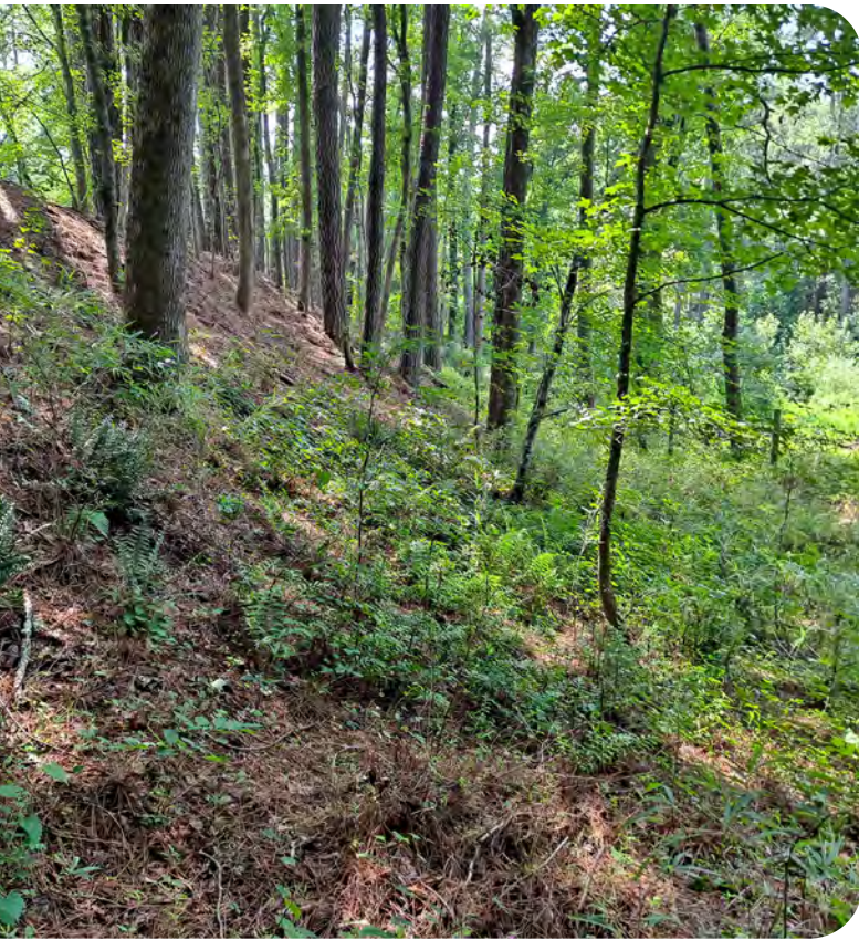
Mature tree growth on the dam of pond number 3
