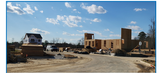
CONSTRUCTION CONTINUES! Forestville Village
