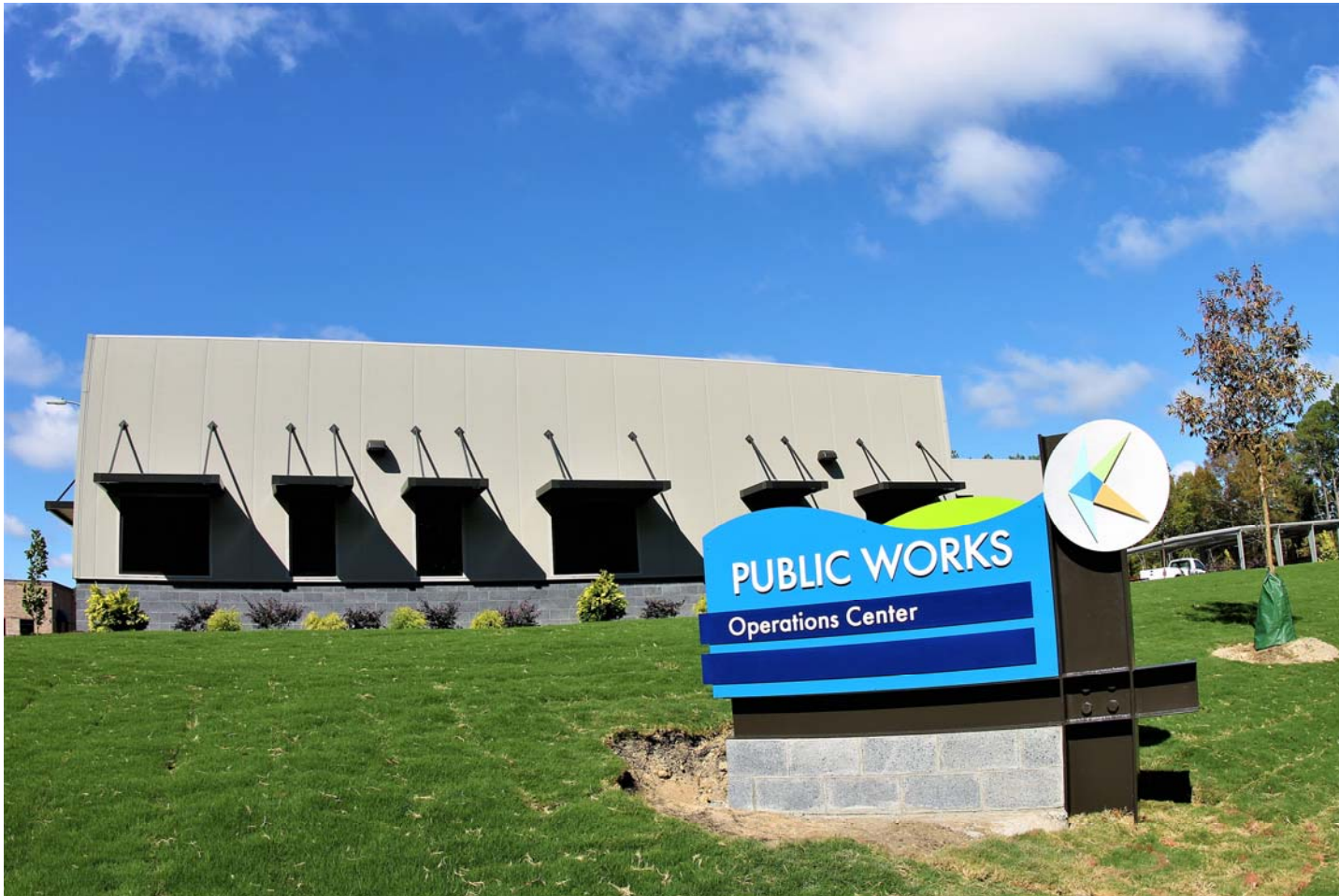
New Public Works Building Opened in Fiscal Year 2020
